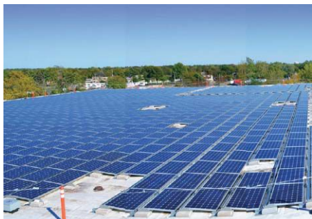
MV Sport/Weatherproof (asi/68318) uses these photovoltaic cells to supply 95% of the electricity it needs at its decorating facility.
